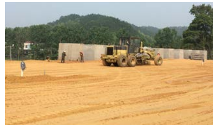
Fig.2 Paving and leveling
